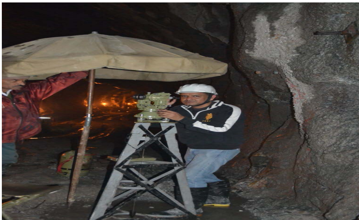
Tunnel Alignment at Punatsang Chhu Hydro Electric Project in Bhutan.
